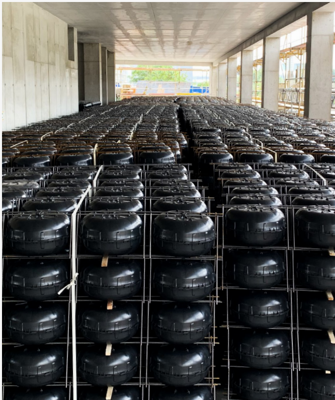
Practical where storage space is limited: Cobiax void formers of the „Cobiax SL“ type are delivered in component parts and can be easily assembled on site to form modular bars. Source: Cobiax, Bielefeld.
